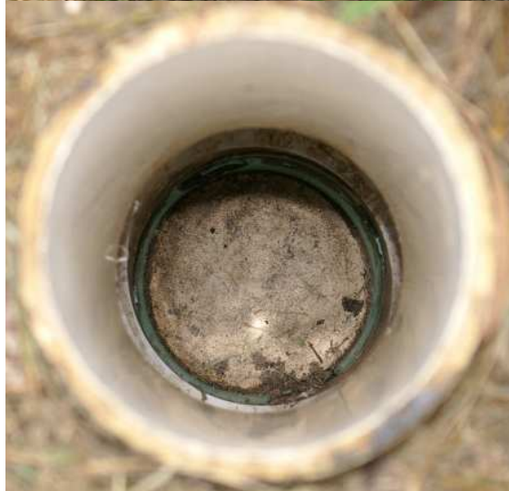
Drainfield dry after installation of VBT™.
